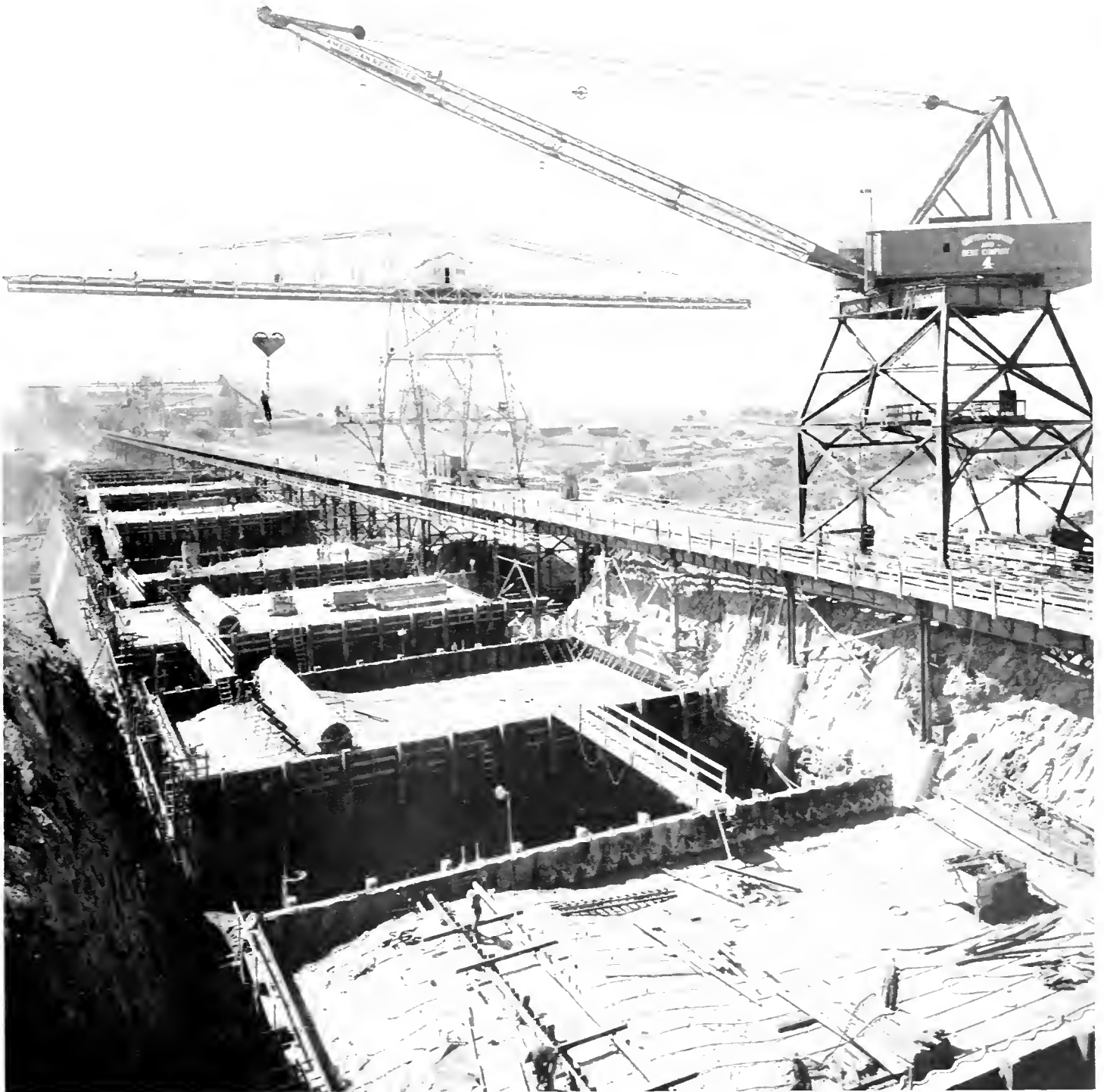
This view of Friant Dam shows the progress of concrete pouring made to date by the trestle and crane system
